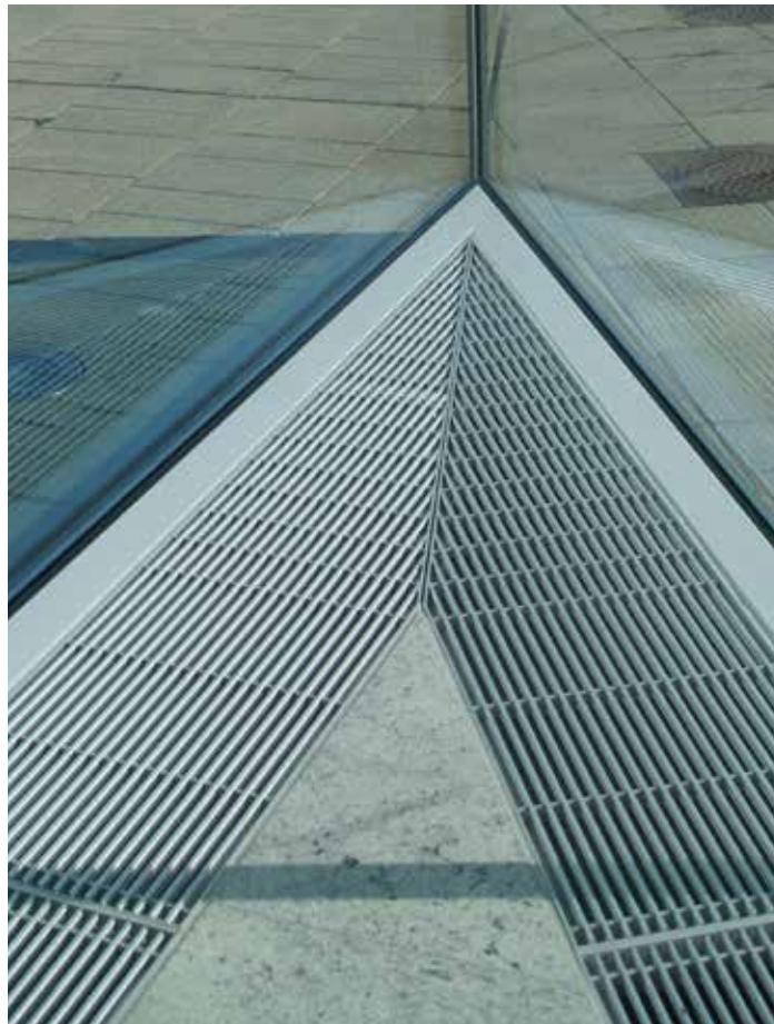
Mini Canal custom made corners (Rigid aluminium grilles) Aller Media Building - Copenhagen Denmark
