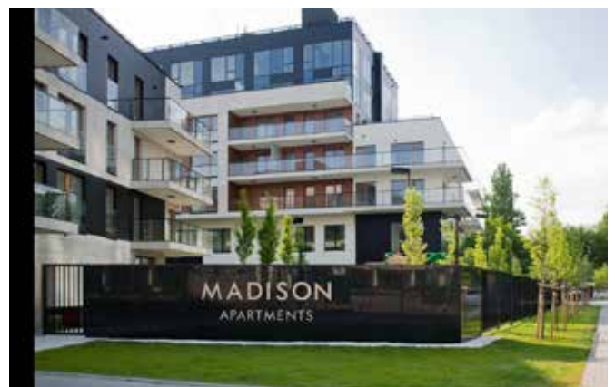
Madison Apartments - Polen - Clima Canal
