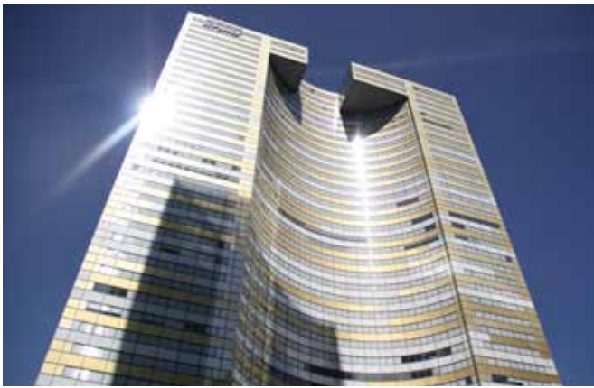
Tour Eqho - France - Clima Canal
